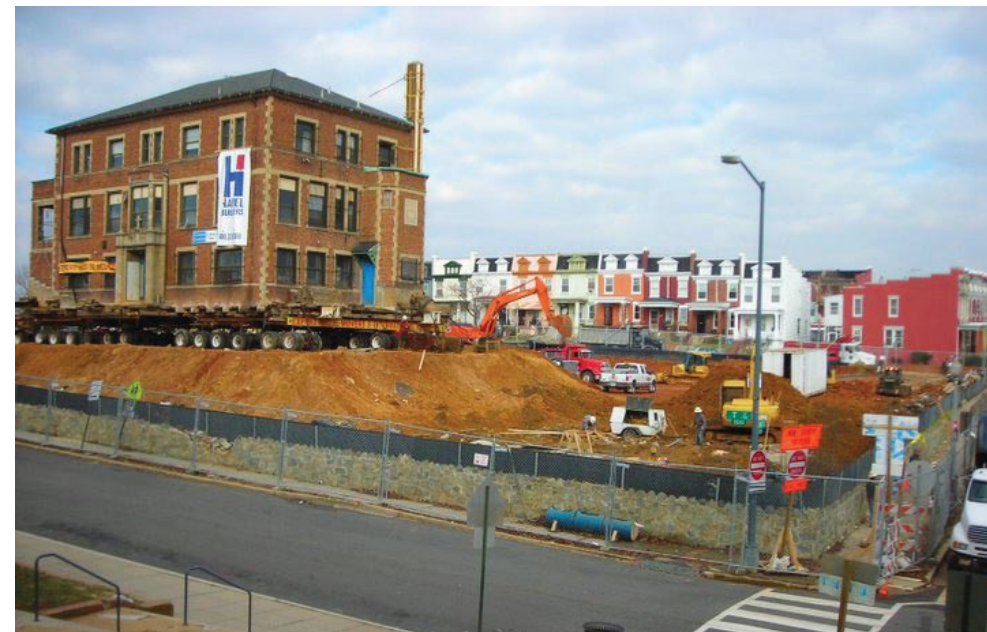
St. Martin's historic convent, which formerly housed nuns who taught at its grammar school, was relocated to serve as the centerpiece of a new Washington, D.C. development.
