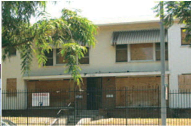
Hayworth House prior to renovation.
