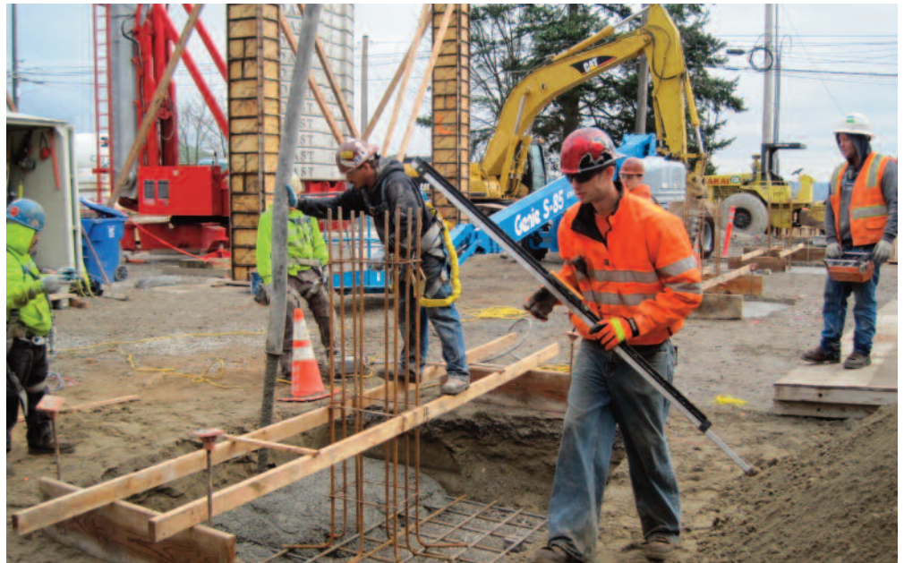
Construction on New Tacoma Senior Apartments.
